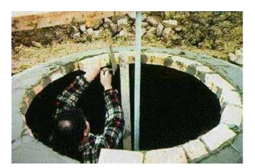
Figure 3: Fixed-dome plant in Tunesia. The final layers of the masonry structure are being fixed.
