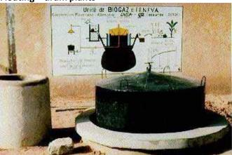
Figure 7: Floating-drum plant in Mauretania
