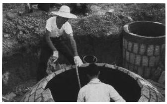
Figure 6: Installation of a Shanghai fixed-dome system near Shanghai, PR China Floating-drum plants
