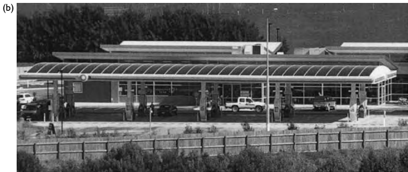
Figure 7.29 Examples of grid-connected photovoltaic installations. (a) An office building at the University of Melbourne, Australia, with an envelope of PVs on its north-facing wall. This building also includes many other features of ‘sustainable design’ – see Section 6.3. [Photo courtesy of University of Melbourne.] (b) A service station in Australia with PVs on its roof. Note the juxtaposition of renewable and non-renewable energy sources. [Photo by courtesy of BP Solar.]
