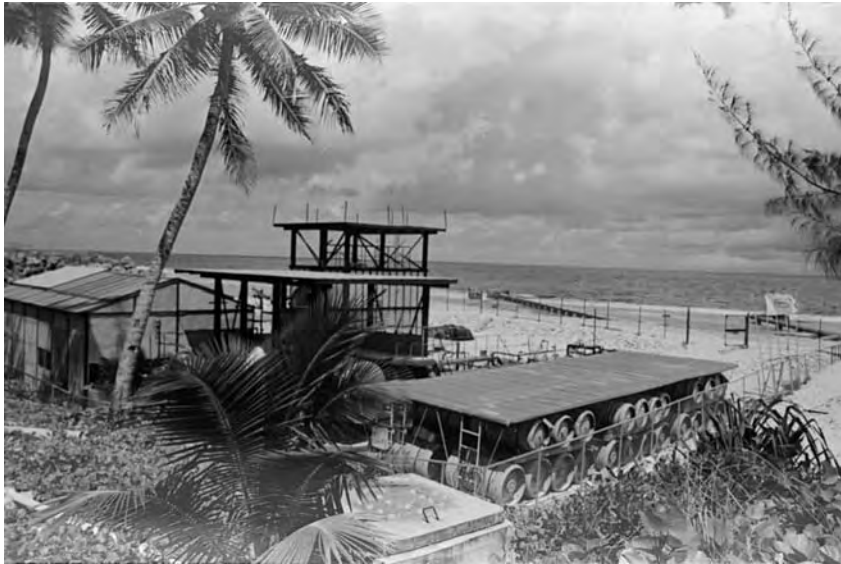
Figure 14.4 Experimental land-based OTEC plant on Nauru, built by Tokyo Electric Power Services Company in 1981 for research. It was a 'closed cycle' system, rated at 100\text{kW}_e output. On the photograph the vertical framework to the rear contains the condenser, the nearer large horizontal cylinder is the evaporator, the turbine house is at the left, the cold water pipe runs out to sea (in the background), and cylinders in the foreground contain spare working fluid.
