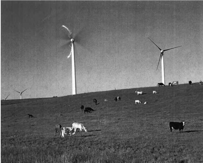
Figure 9.29 A wind farm in Minnesota, USA, with agricultural activity continuing underneath. [Photo by Warren Gretz, courtesy of [US] National Renewable Energy Laboratory.]
