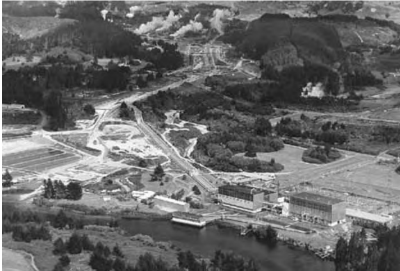
Figure 15.9 The Wairakei geothermal power station in New Zealand. Well-heads are at top of photo; condensed steam is discharged into the Waikato River at bottom. [Photo by courtesy of Contact Energy, New Zealand.]
